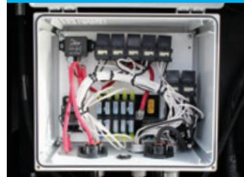
Electrical relays & fuses are protected from the elements in a sealed NEMA 4 enclosure. The wiring is heat stamped with numbers for easy identification.
