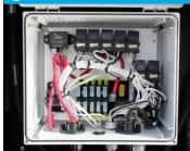
Electrical relays & fuses are protected from the elements in a sealed NEMA 4 enclosure. The wiring is heat stamped with numbers for easy identification.
