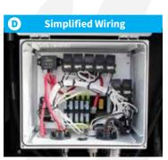
Electrical relays & fuses are protected from the elements in a sealed NEMA 4 enclosure. The wiring is heat stamped with numbers for easy identification.
