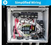
Electrical relays & fuses are protected from the elements in a sealed NEMA 4 enclosure. The wiring is heated stamped with numbers for easy identification.
